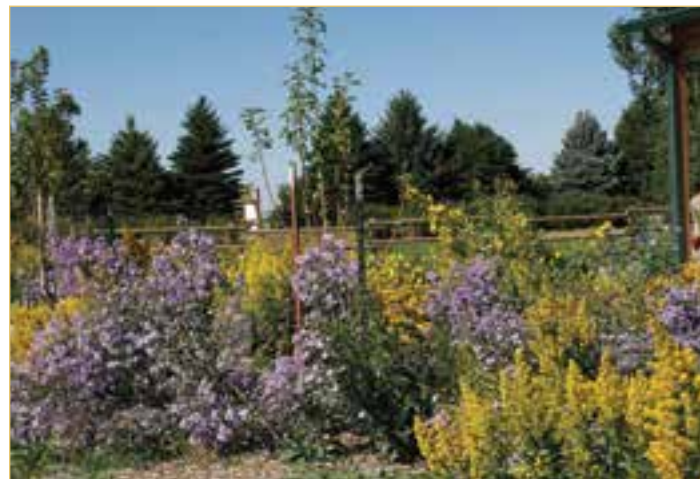
The newly constructed Horticulture Farm Barn, with a surrounding rain garden. The rain garden was designed and installed by Jennifer Britton's Horticulture 336 class.
